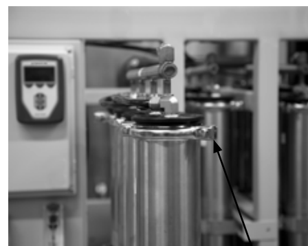
FIGURE 81-1: DRISTEEM REVERSE OSMOSIS MEMBRANES
